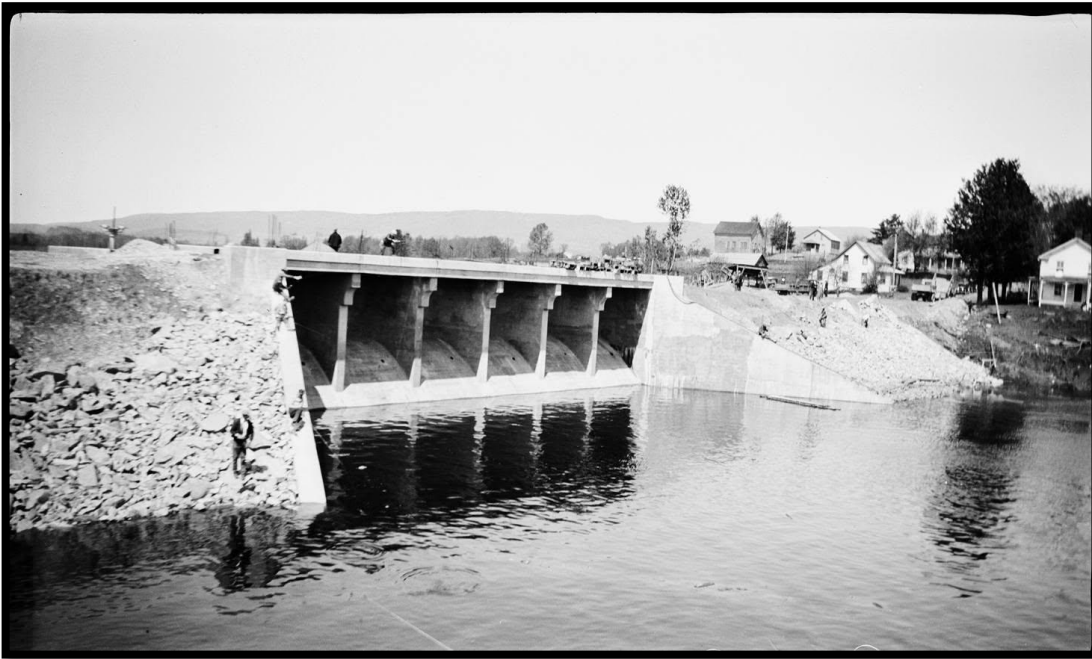
The new bridge, Spring 1931. Courtesy of Paul Larner, from the H.A.Phelps collection.
