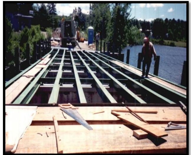
Replacing the deck of the bridge, 1991
