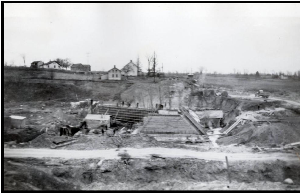
Construction of the Dam and Bridge, 1931. Courtesy of Bruce Becker.
